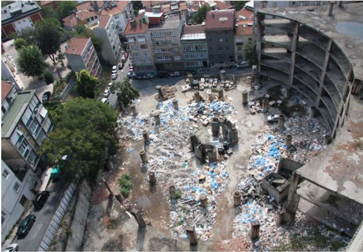
Park Hotel, view from rooftop
